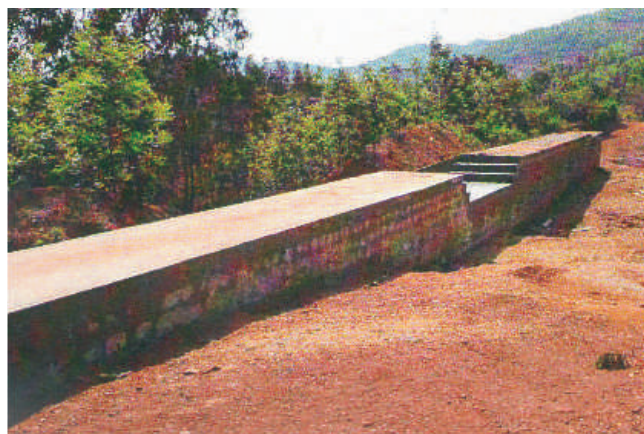
Check Dam Constructed on a mine site.
