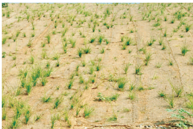
Geotextile method adopted for plantation on slop of waste dump at Rampura Agucha lead zinc mine of M/s HZL in Bhilwara district.
