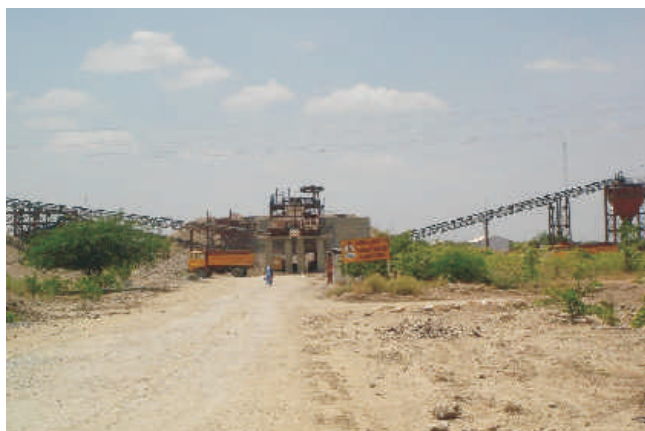
Kankar screening plant to remove silica in Marvarperungudi limekankar mine of M/s Madras Cement Limited, R.R. Nagar in Tamilnadu State.
