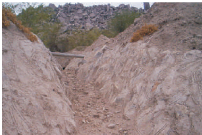
Garland Drain along the waste dump road at Rampura Agucha lead zinc mine of M/s HZL in Bhilwara district.
